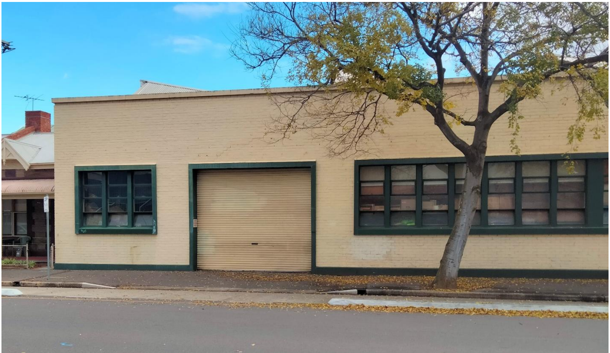
Photo 3.2 – Existing crossover on Regent Street North
