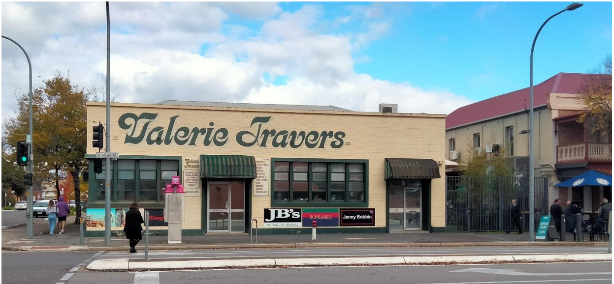
Photo 3.4 – Adjoining residential dwellings to the south
